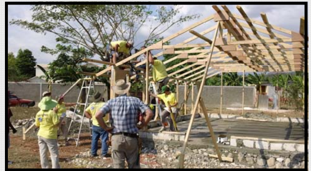
A new Church being built in Haiti
